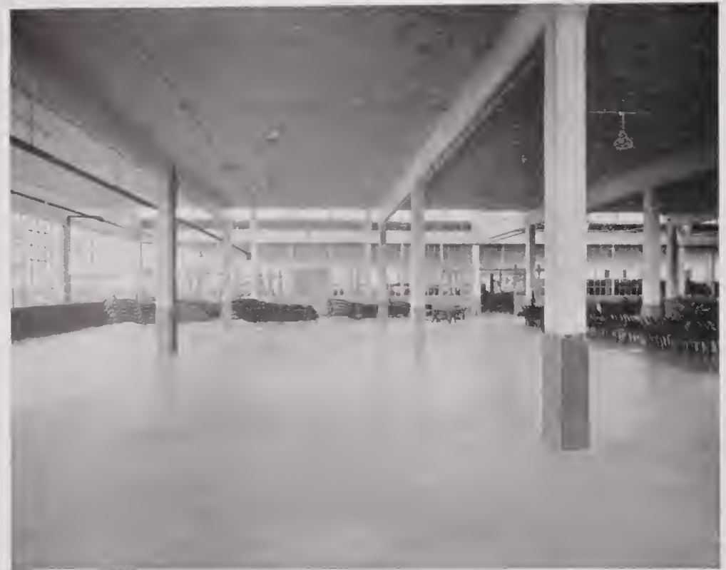
CONCRETE FLOORS PAINTED TO PREVENT DUST
